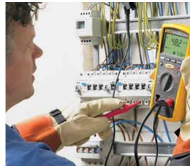
Insulation Test at a distribution Panel
